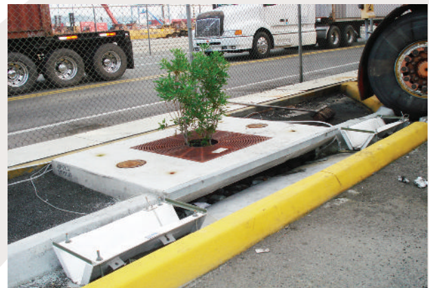
Filterra® monitoring unit at an industrial port.
