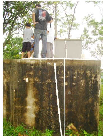
Chlorinator installation above the water tank
